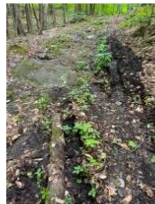
Steep, rocky sections compromise vehicle passage.
